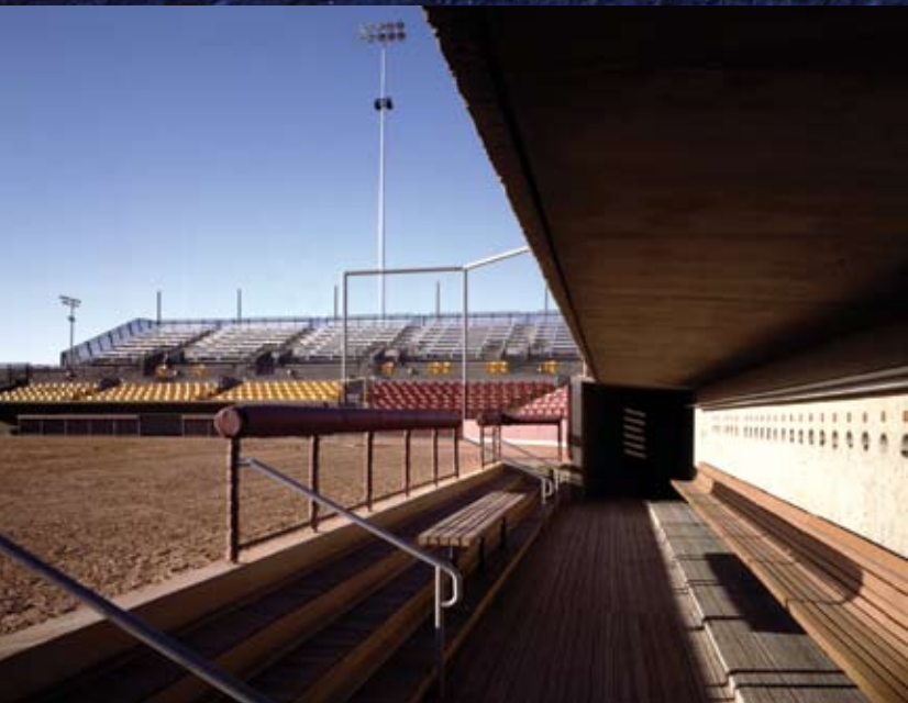
| P.212 | JONES STUDIO INC | ARIZONA STATE UNIVERSITY WOMEN'S SOFTBALL STADIUM | 1999 | 1,500 SEATS | GALVALUME CLADDING |
