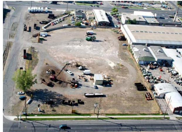
Construction of Artspace Commons.
