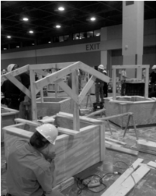
Figure 6: Planter boxes under construction at Arizona Skills USA Construction Competition. Photograph by Braden Kay.
